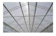
Specifically for LEXAN THERMOCLICK 40 and 50 mm sheet, a new aluminum profile system with an especially designed cold bridge connection is developed . This new system prevents manifestation of condensation in the inside of the profile for partition walls, floor, ceiling and roofing.
